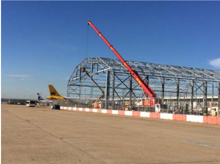
Figure 1. An 'on airport' development in progress
