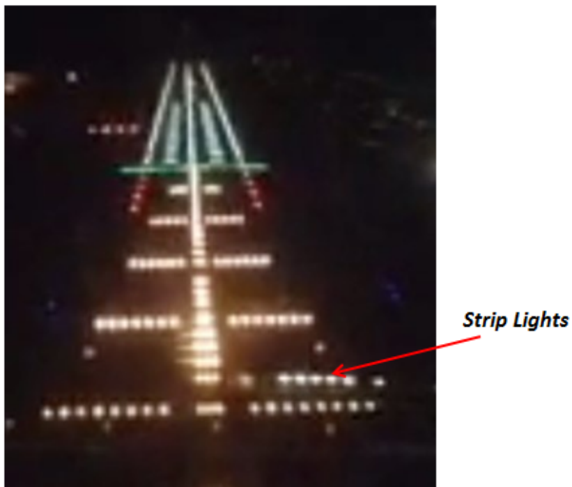
Figure 4. Five strip lights which are causing confusion within the runway approach lights
